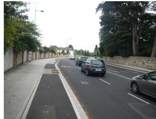
Manholes in cycle lane/track
