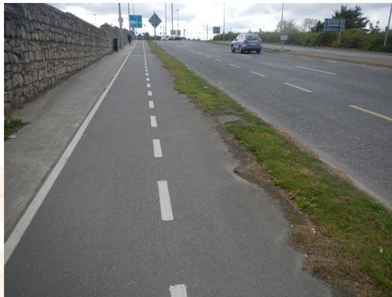
Grass encroaching onto cycle facilities
