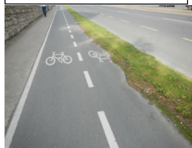
Grass encroaching cycle facilities
