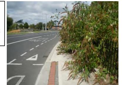
Shrub is encroaching on footpath resulting in pedestrians walking into cycle lane which may result in a cyclists/pedestrian collision. Cut back vegetation.
