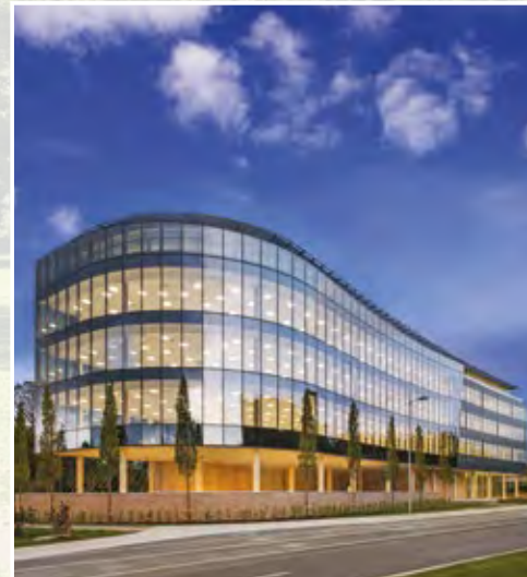
South County Business Park
