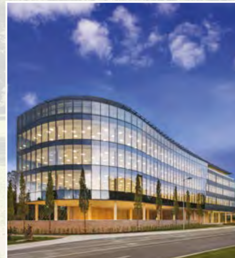
South County Business Park
