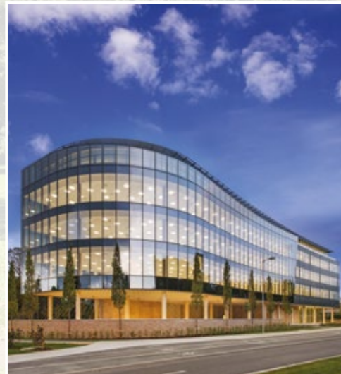
South County Business Park
